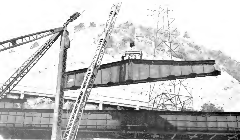
This 70 ton member had to be swung 100 feet in the air
